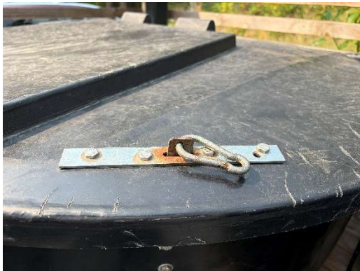
Example 2: Slotted Metal 'Pin' with Locking Carabiner
