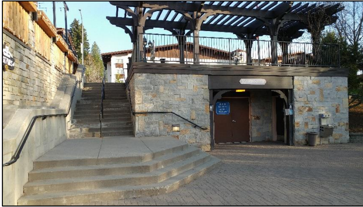
Front Street Side of Restroom Facility
